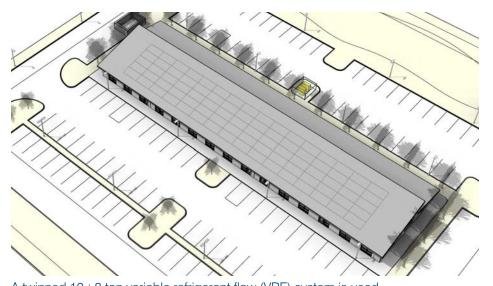
A twinned 10+8 ton variable refrigerant flow (VRF) system is used for heating and cooling. The units are located on grade behind the building. Additional trees have been planted on the north, east and west facades to reduce solar heat gain on the building.
